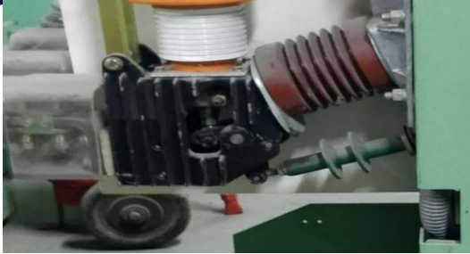
FIG 12 INSPECTION OF VACUUM LEVEL
