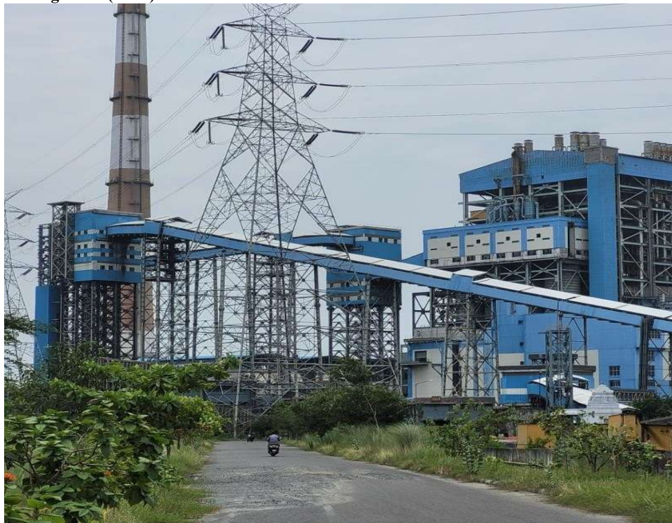
Figure 1: Coal handling plant
