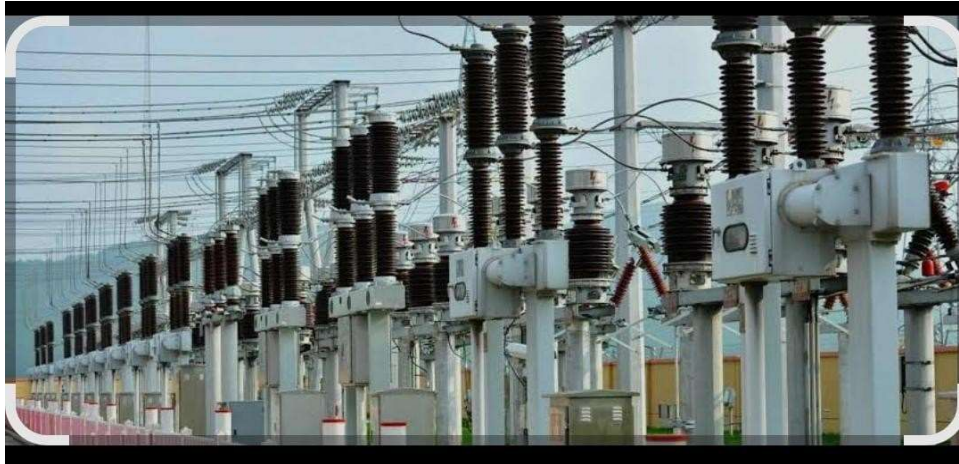
Figure 9: Lightning Arrester
