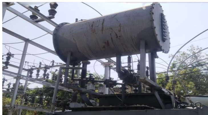
Fig 2 : Conservator tank
