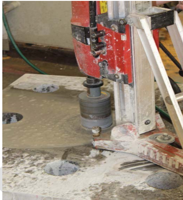
Figure 4. Removal of core borehole from concrete slab
